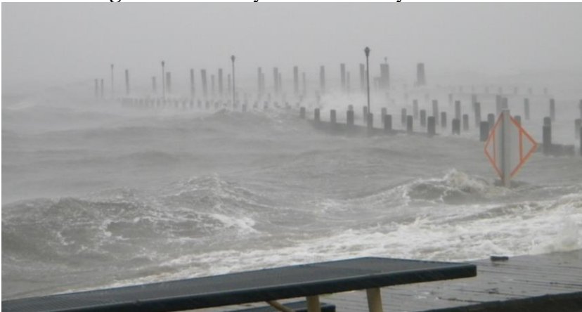
Figure 10: Destroyed Dock at Bryant Park
