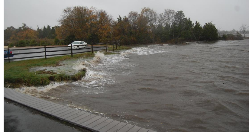
Figure 14: Flooding at the Bay-End of Tuscarora Avenue
